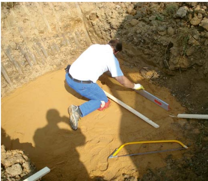
Fig. 3a Foundation pit with sand bed
