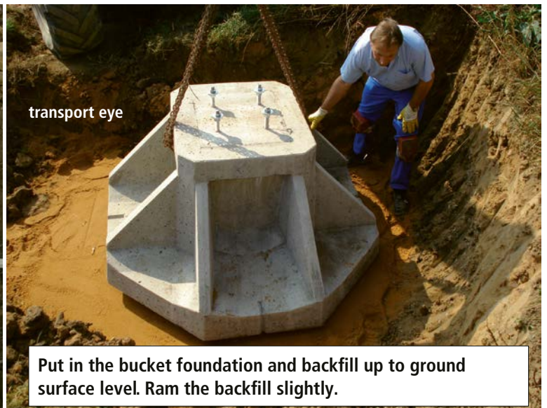
Fig. 3b Bucket foundation I
